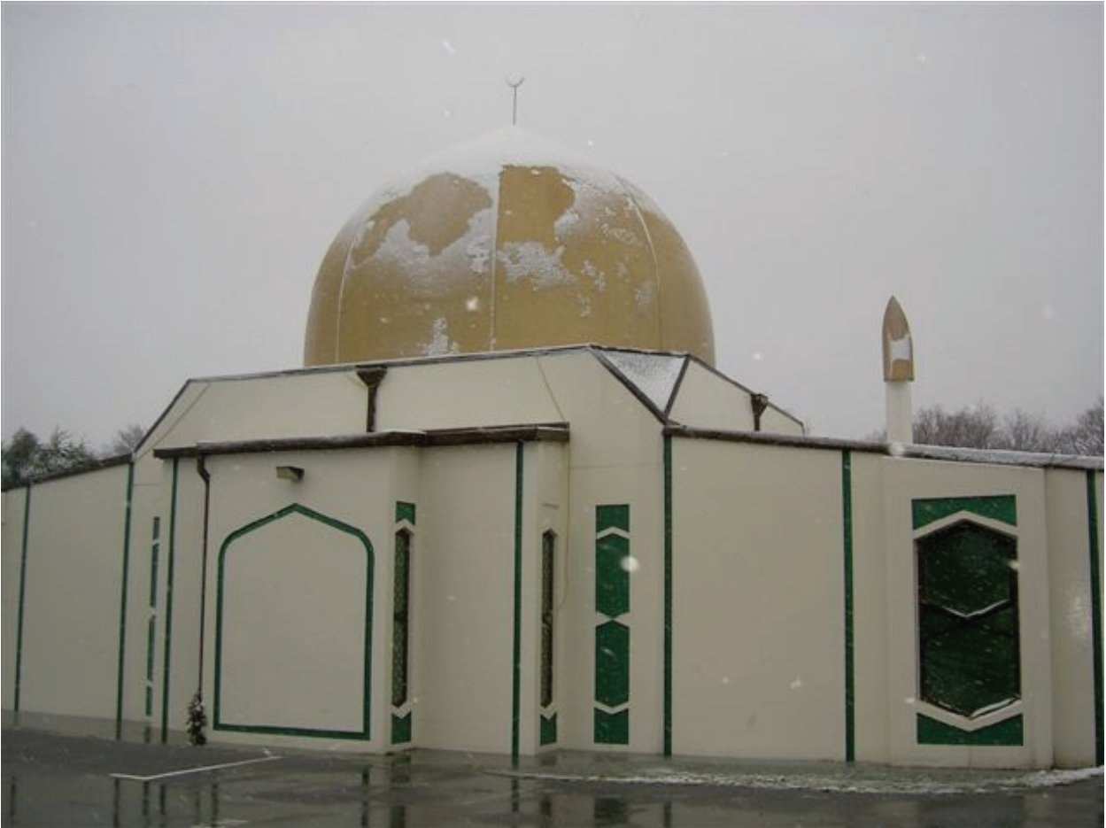
CANTERBURY MOSQUE, NEW ZEALAND
