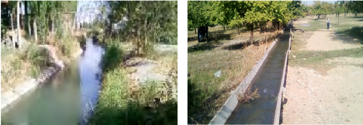
Figure 3. View of the concrete covered part of the Ak-Tatyr canal – the intra-farm part of the canal (left photo) and view of the tray section of the Jaiylma canal (right photo)
